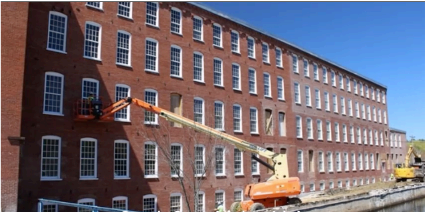
Construction underway at the China Mill rehabilitation project using 79-E in Allenstown, NH. (Image via allenstown-alt.com )
