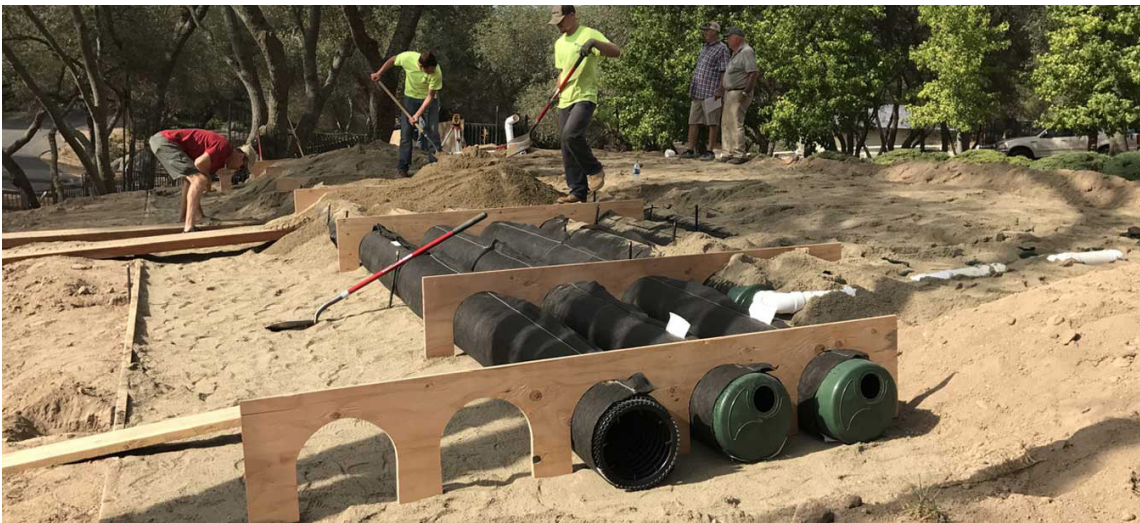
Installation of the municipally owned Blodgett Landing community septic system in Newbury. (Images via NextGen Septics)
